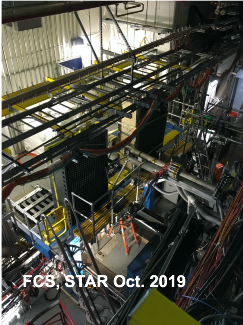
Figure 90: A view of the installed forward ECal detector halves, left and right from the beam pipe.
